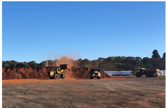
Figure 2: Bauxite loading from ABx's port stockpile
