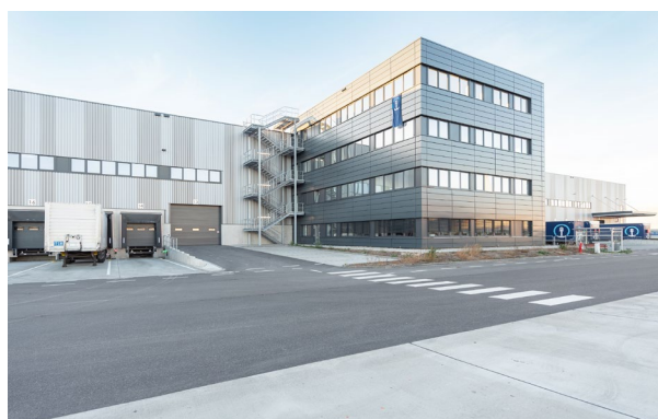
Goodman Hamburg III Logistics Centre, Hamburg, Germany
