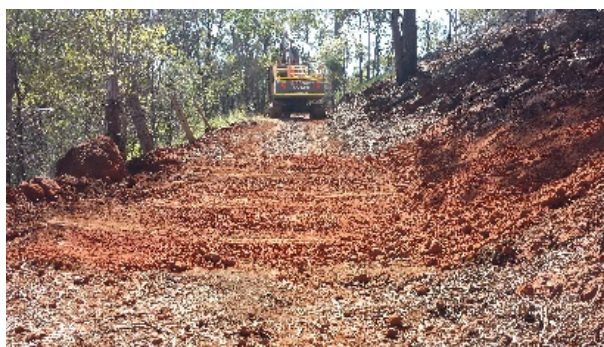
Figure 4: repaired site of pit BJP001 on forest track
