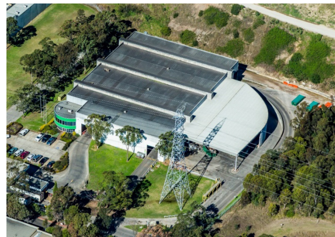
Davis Road Waste Transfer Station, Wetherill Park NSW
