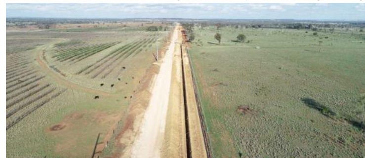
Example of pipeline installation
