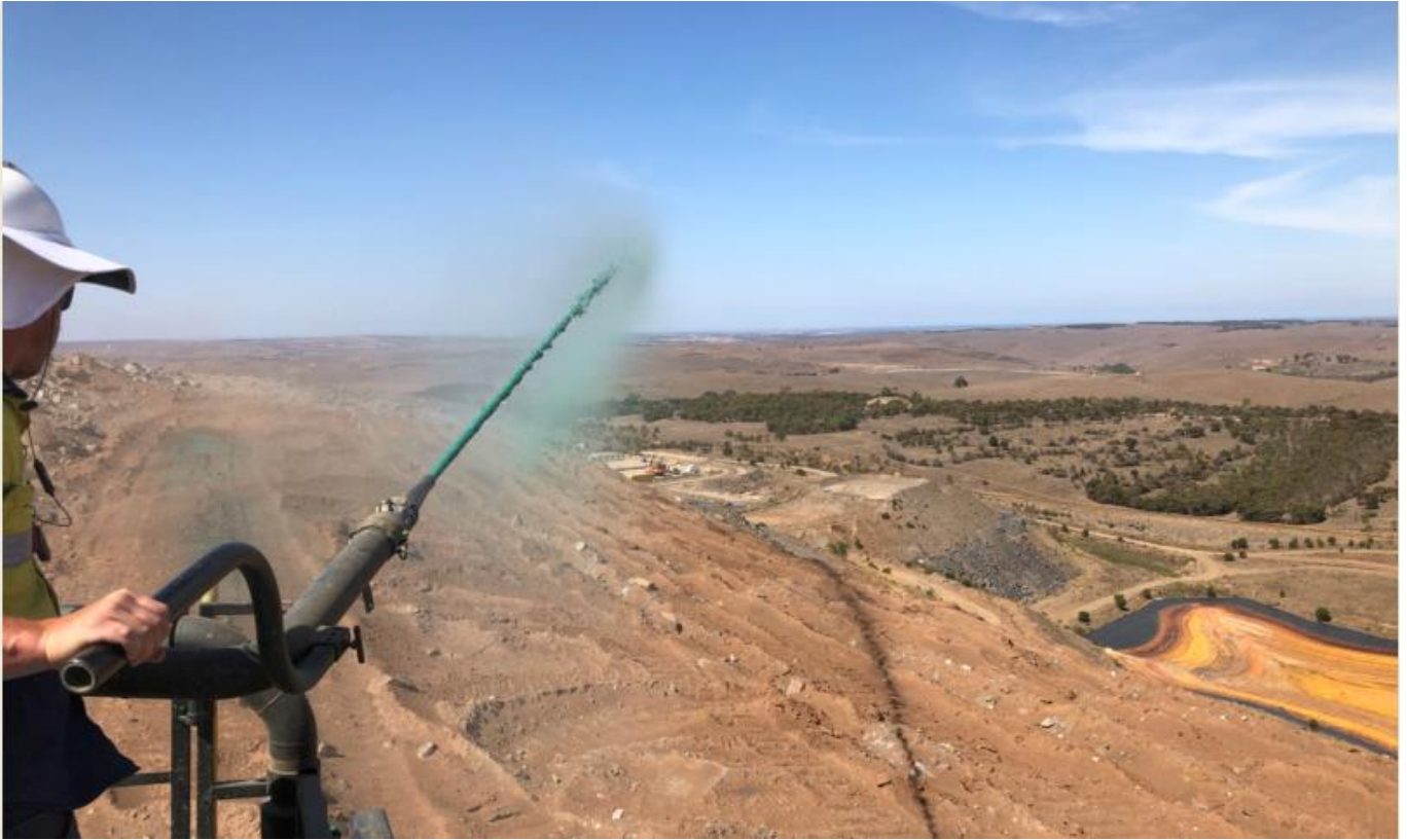
FIGURE 4. REHABILITATION – HYDROSEEDING
