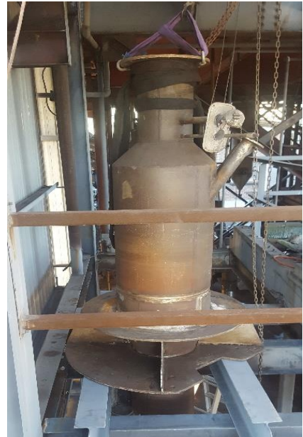
Installing the upper body of enhanced FB Roaster
