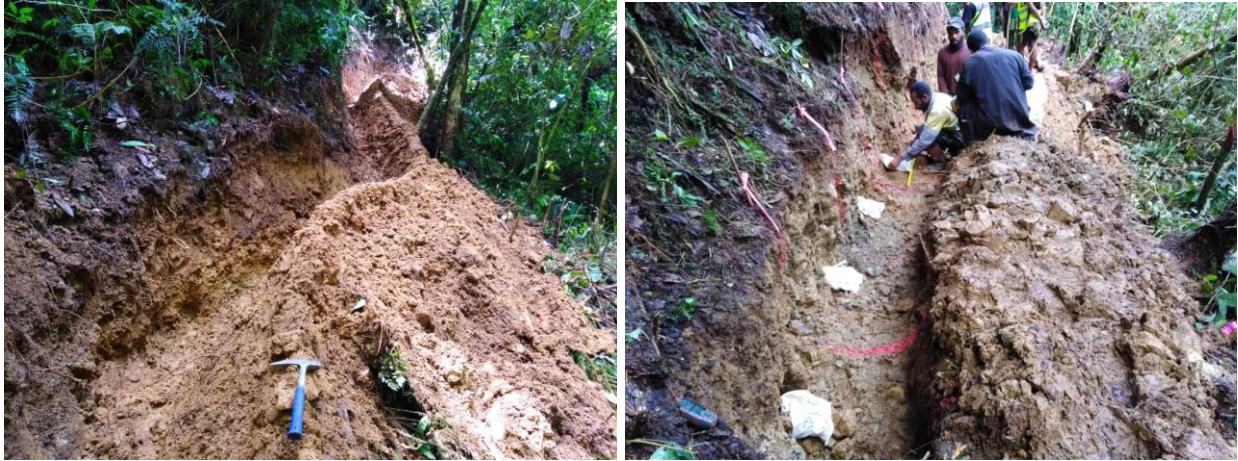
Figure 2: Trenching Activities at Mongae Creek
