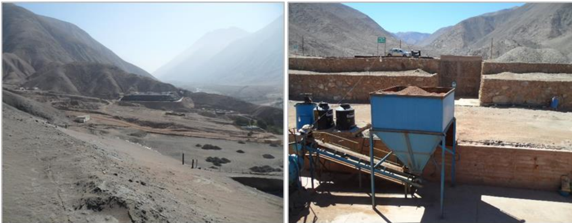
Photo 5 & 6: “Existing Infrastructure: Chimu Gold Plant”
