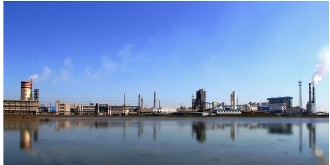
CNE steel mill
