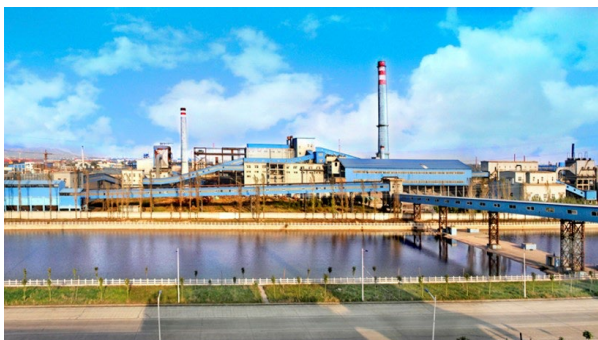
CNE steel mill
