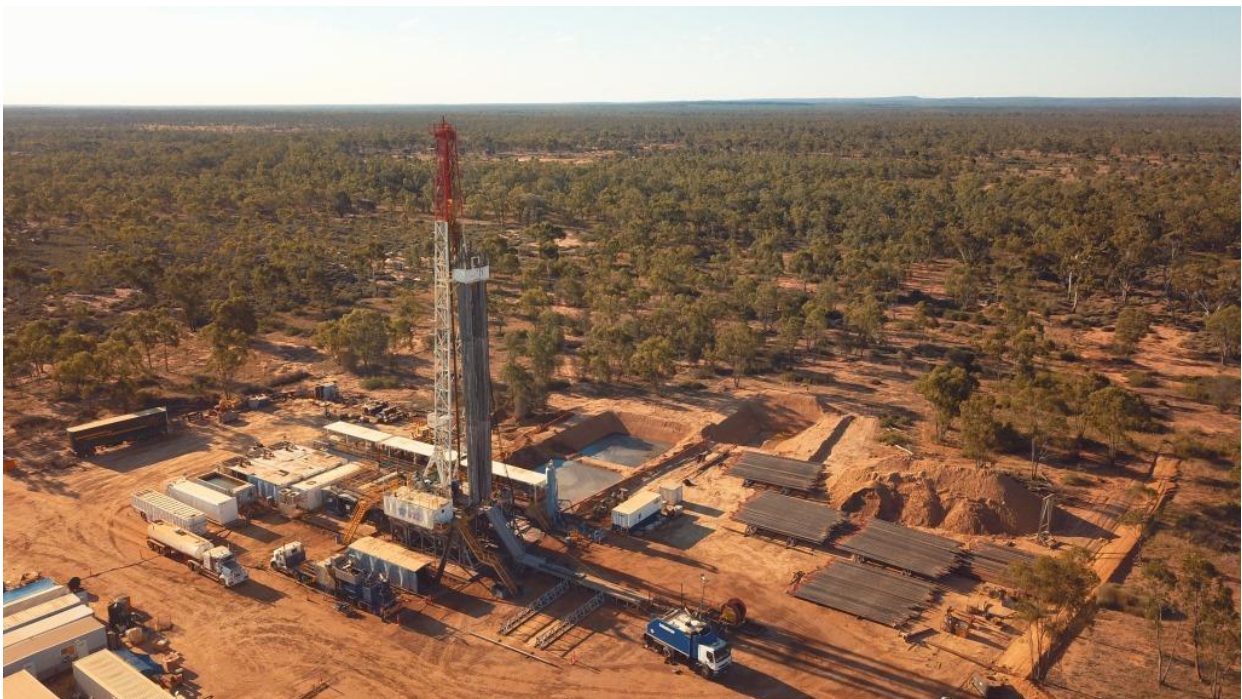
Figure 1 – Ensign Rig 932 on site at Albany 2
