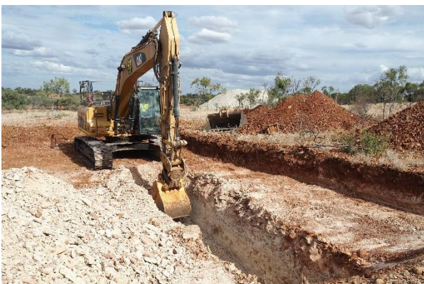
CAPTION: Excavator “free-digging” near surface phosphate rock at Ardmore for bulk samples.
