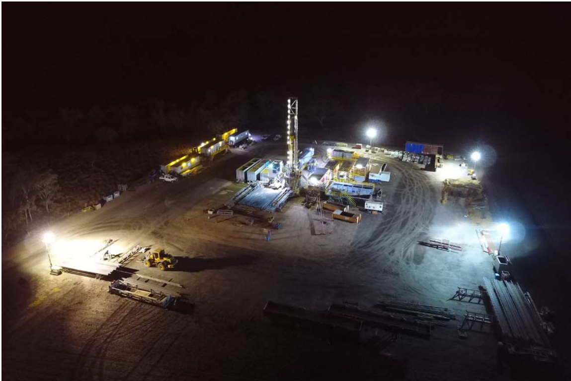
Ensign drilling rig 964 on location of the Armour Energy Myall Creek 4A well June 2018
