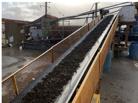
Mill feed at Granville Processing Plant
