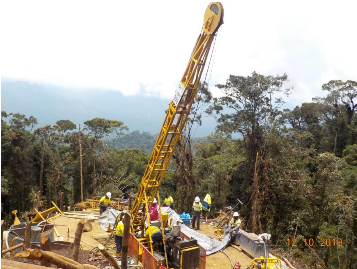
Figure 2: Drill rig set-up as of 12 October.
