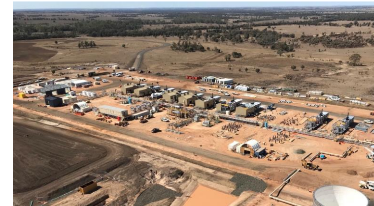
Project Atlas gas processing facility; 15 PJ/year (40 TJ/day including 8 TJ/day installed redundant capacity), expandable to 18 PJ/year (48 TJ/day)
