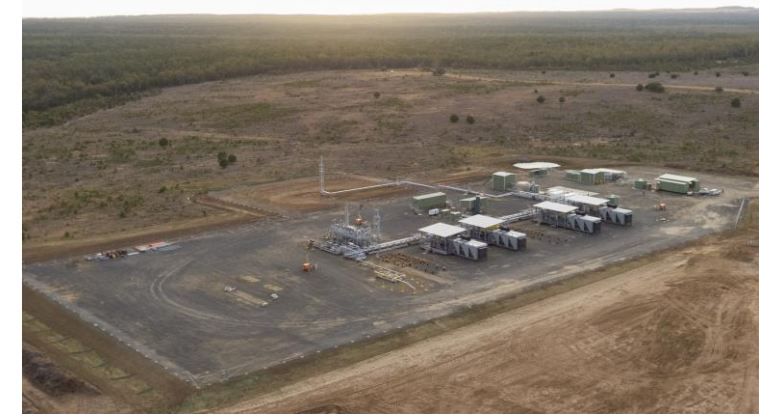
Roma North gas processing facility; 6 PJ/year (16 TJ/day) initial capacity, expandable to 18 PJ/year (48 TJ/day)
