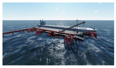
The jetty design simplifies and de-risks the construction process which previously comprised several interdependent stages. The marine and land-based construction can now proceed concurrently until the final stage when the conveyor and loader are to be installed on the suspended deck and pontoon. In order to avoid the need to dredge to the required depth for woodchip vessels, the jetty
