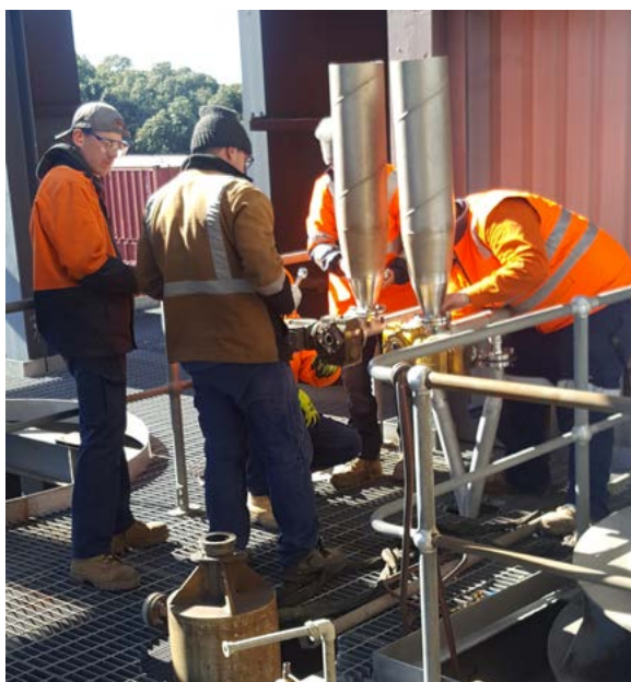
Installing the pellet and feed hoppers on the FBR
