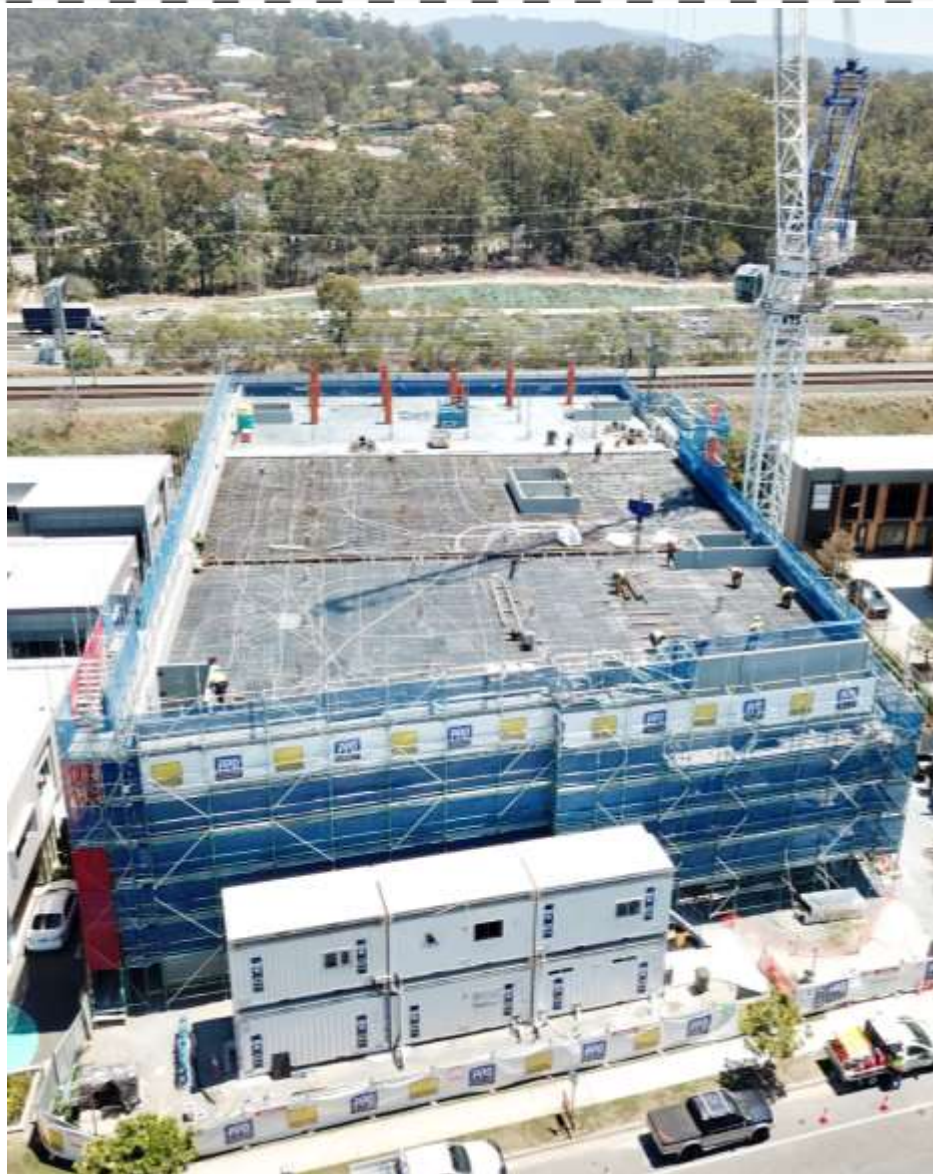
National Storage Robina expansion underway
