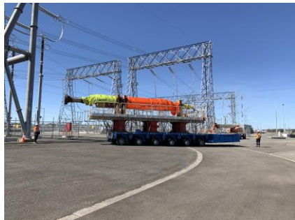
Old rotor being removed at Mortlake
