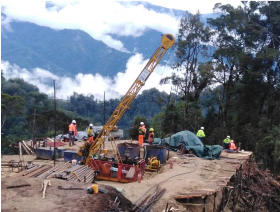
Figure 3. Drill Rig set up on MCD004
