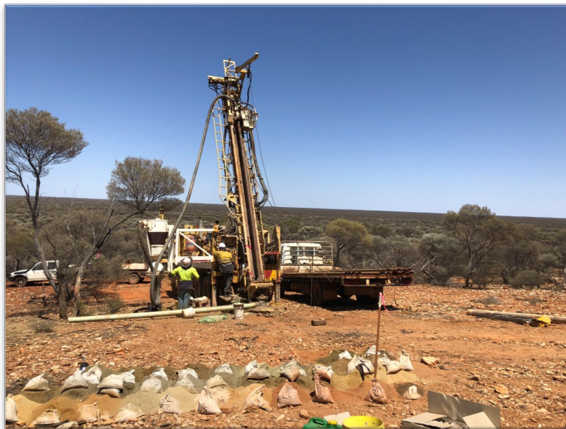
Plate 1: RC Drilling at Creasy 1
