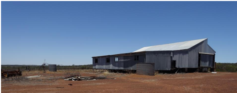
Shearing Shed Bundybunna November 2019
