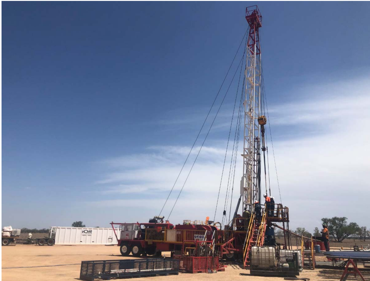
Figure 2 – SWS Workover Rig on Myall Creek 5A location, 29 November 2019
