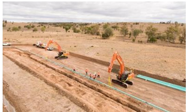
60 km Atlas pipeline completed in October 2019
