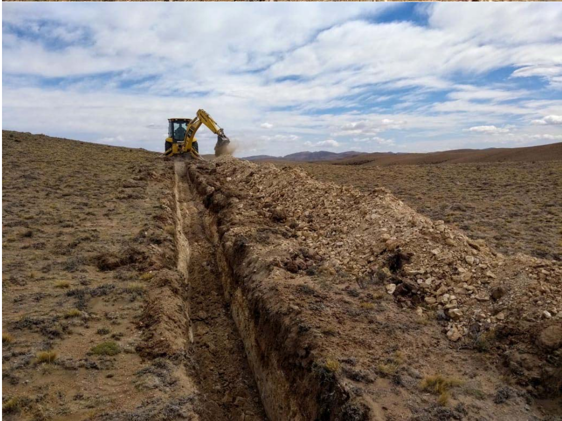
Figure 3 – Trenching at Cachi Gold Project which has exposed the extension of known surface vein systems under soil and ash cover.
