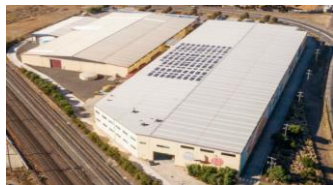
$22.8m (July 2019) 75-95 & 105 CORIO QUAY ROAD, NORTH GEELONG, VIC
