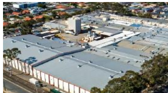
$24.4m (July 2019) 23-41 GALWAY AVENUE, MARLESTON, SA
