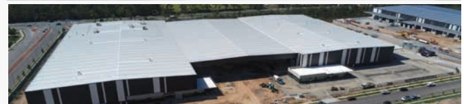
2020 Underway Developments 4 facilities totaling $167m
