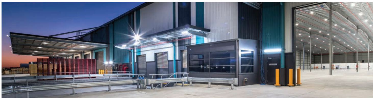
50 Old Wallgrove Road, Eastern Creek
