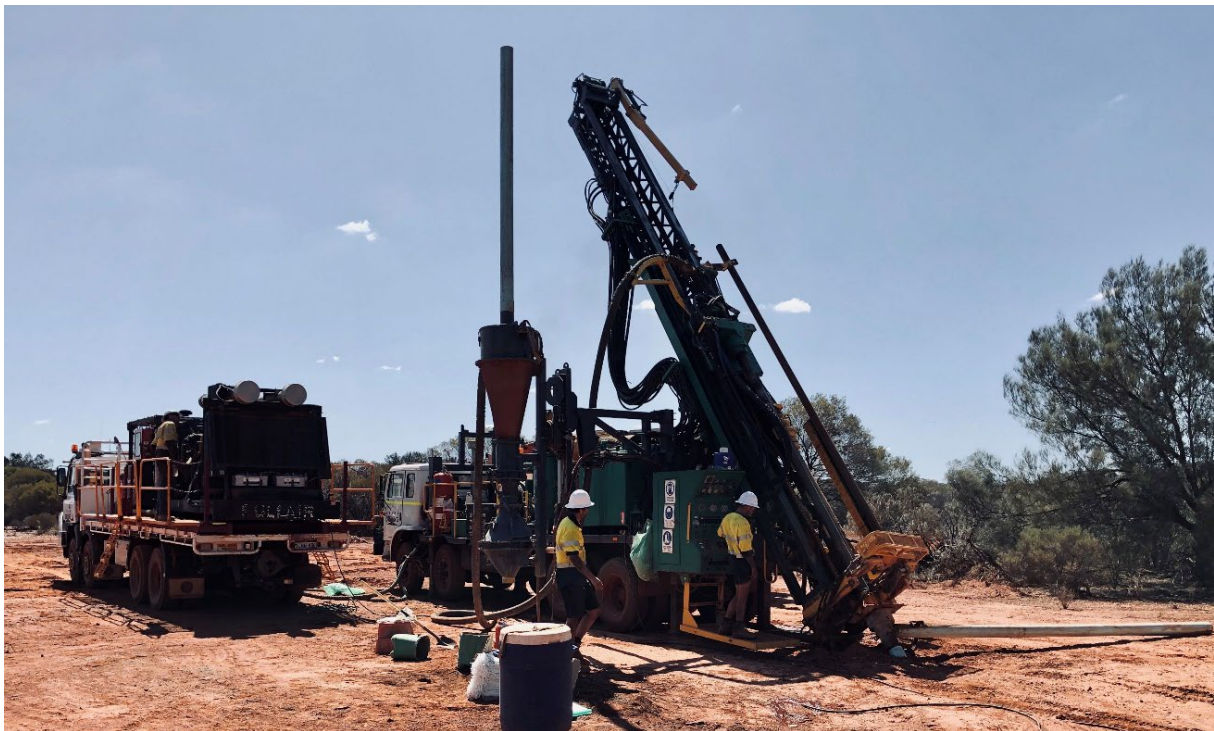
Figure 1: RC Drill Rig commencing drilling the first hole at Metzke's Find.
