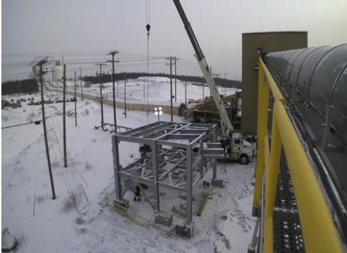
Reclaim conveyor structure assembly ongoing
