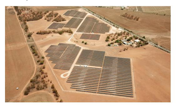
The grid-connected 6.8MW<sub>DC</sub> Mannum Solar Farm Project is owned by a wholly owned subsidiary of Canadian Solar and comprises approximately 17,000 solar panels and utilises single axis tracking technology. The tracking technology facilitates the movement of the solar panels to track the sun during the day, thereby maximising the power output of the solar farm.
