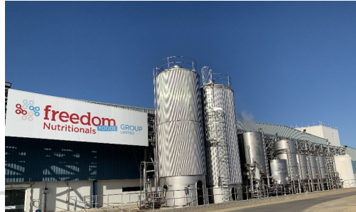
Integrated Nutritional Facility in Shepparton
