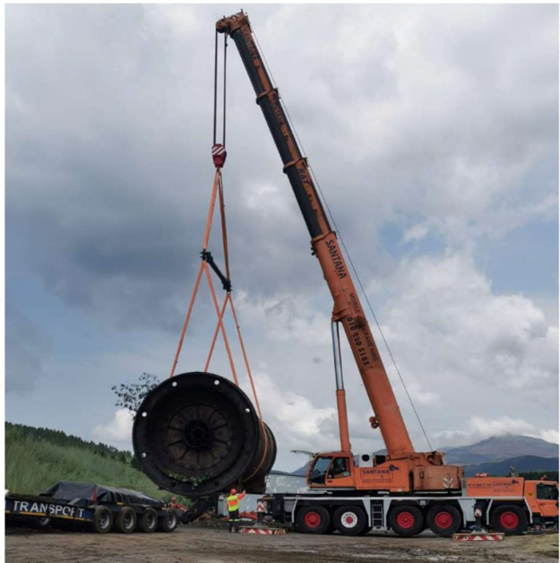
Figure 2: Ball Mill drum being offloaded upon arrival at Theta Gold's TGME CIL Plant site
