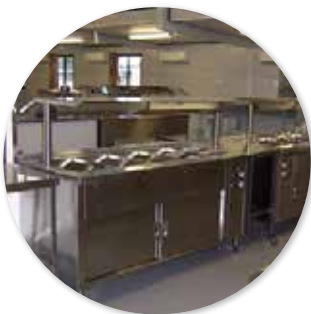
Kitchen & preparation areas
