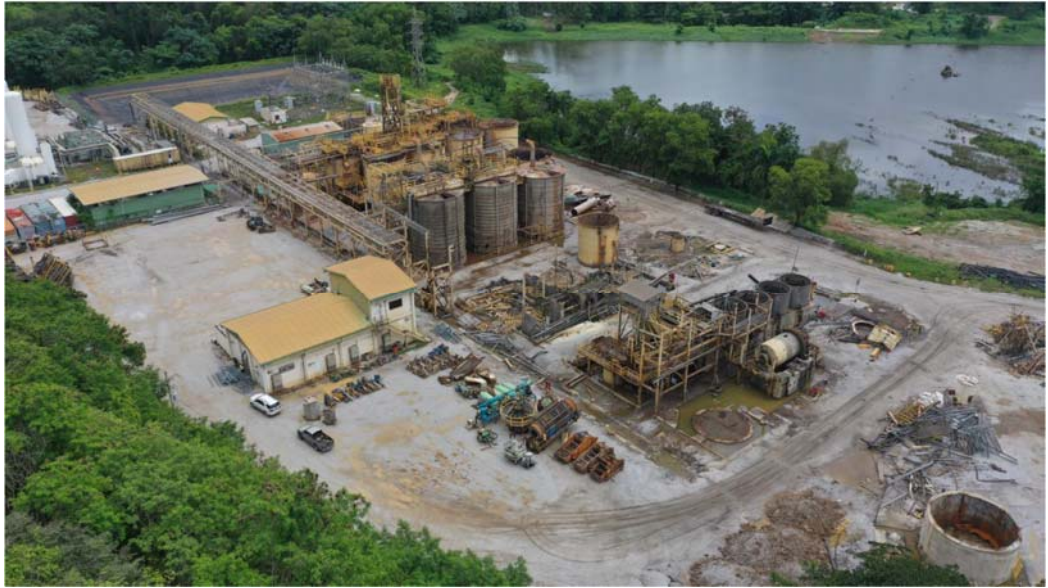
Process plant dismantling
