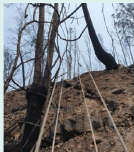
Batemans Bay communications tower
