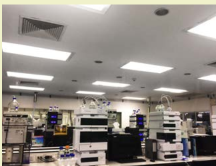
Life Sciences, Perth. LED lighting
