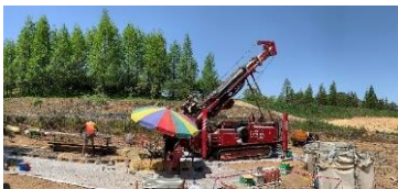
Shin Adit, Deokon – Drilling completed
