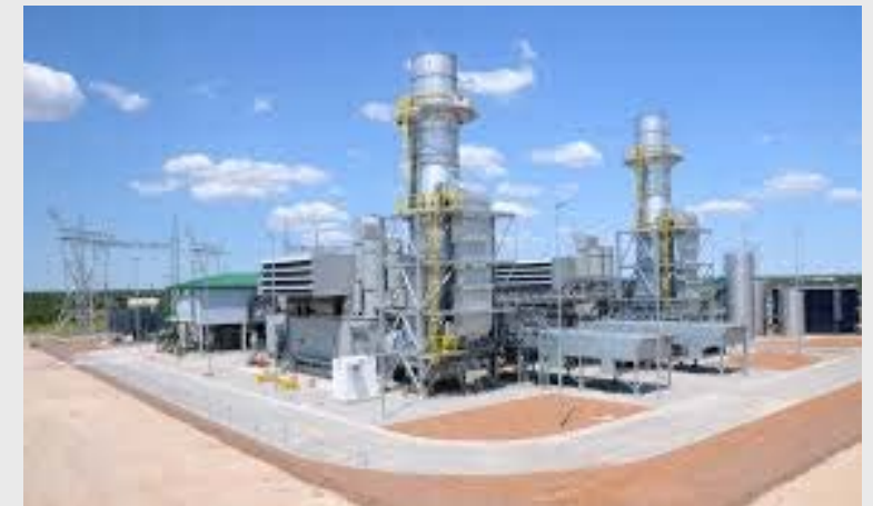
Orapa 90 Mw dual fuel power station
