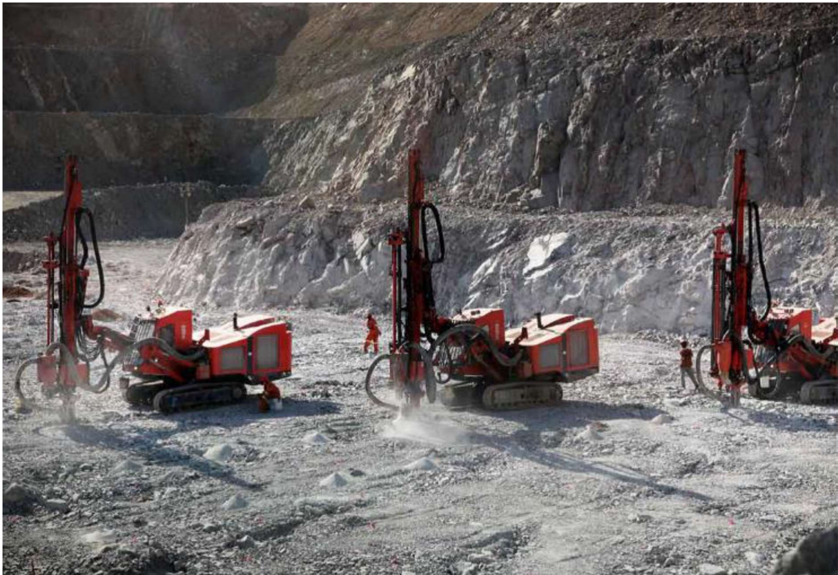
Figure 2: Digmin - Production Drilling at New Luika Gold Mine Tanzania for Shanta Gold
