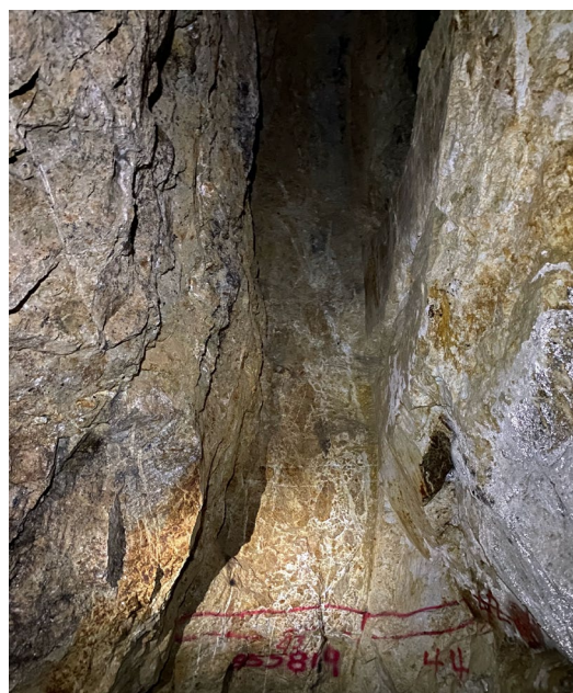
Photo 2 Significant stope on the Apolonia Vein at the future drill target at San Manuel Mine.
