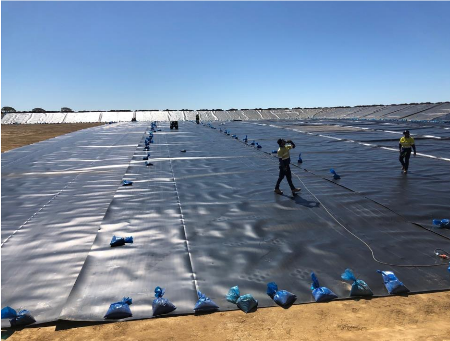
Figure 4. Installation of the liner on the irrigation dam.
