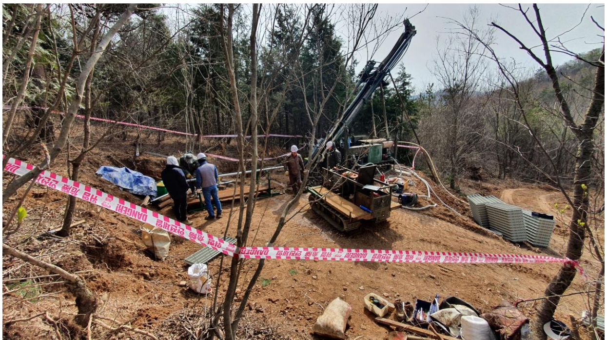
Photo 5 - BPDD015 drill site at 'Spider' looking south-west
