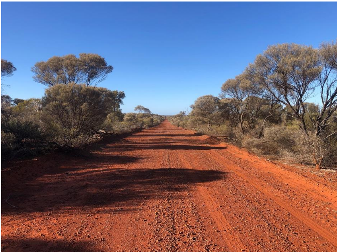
Figure 4: Photo looking north of the ~75km long haul road at Illaara
