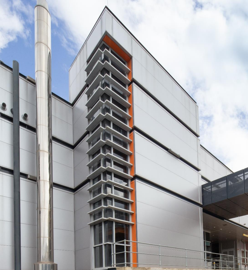
TELSTRA DATA CENTRE COMPLEX, CLAYTON VIC
