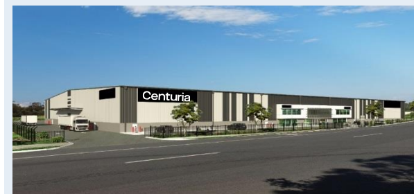
42 HOEPNER ROAD, BUNDAMBA, QLD
