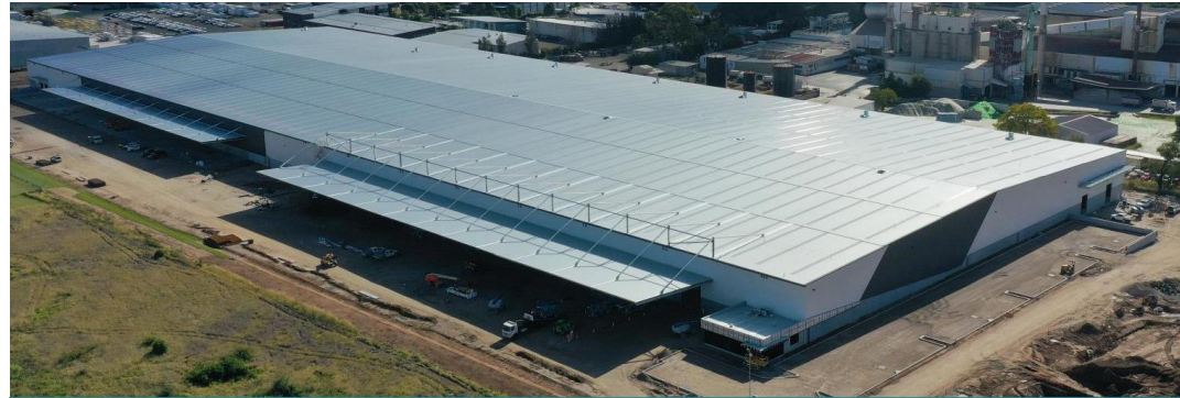
128 Andrews Road, Penrith, NSW
