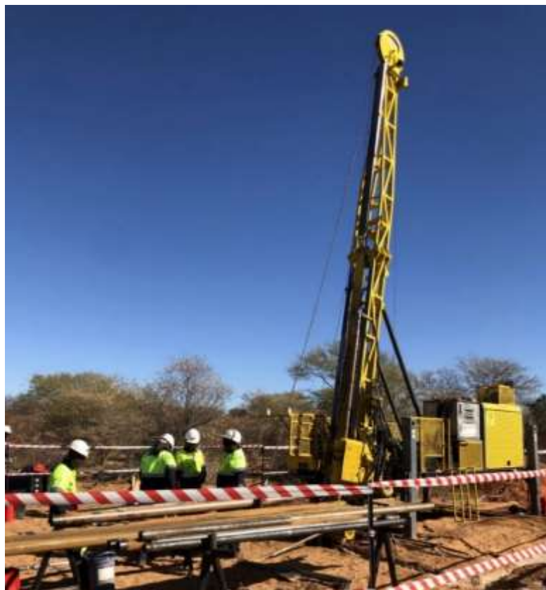
Figure 1: Recent KML drilling operations
