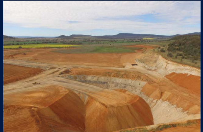
July 2020 final stages of backfilling & topsoil spreading
