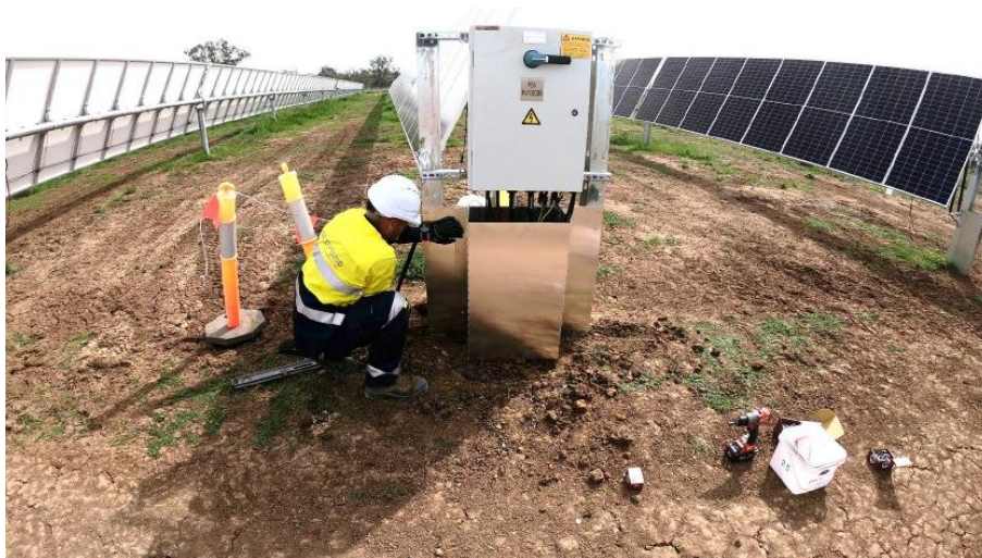
Figure 2. Jemalong Solar Project Panel Installation
