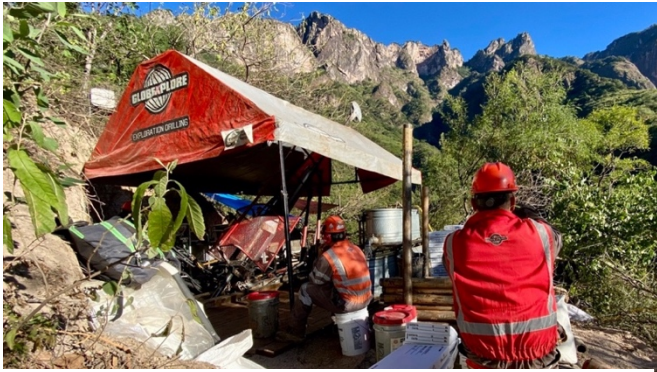
Figure 1 Drilling hole CDH-037 at the La Soledad target, Cometa
