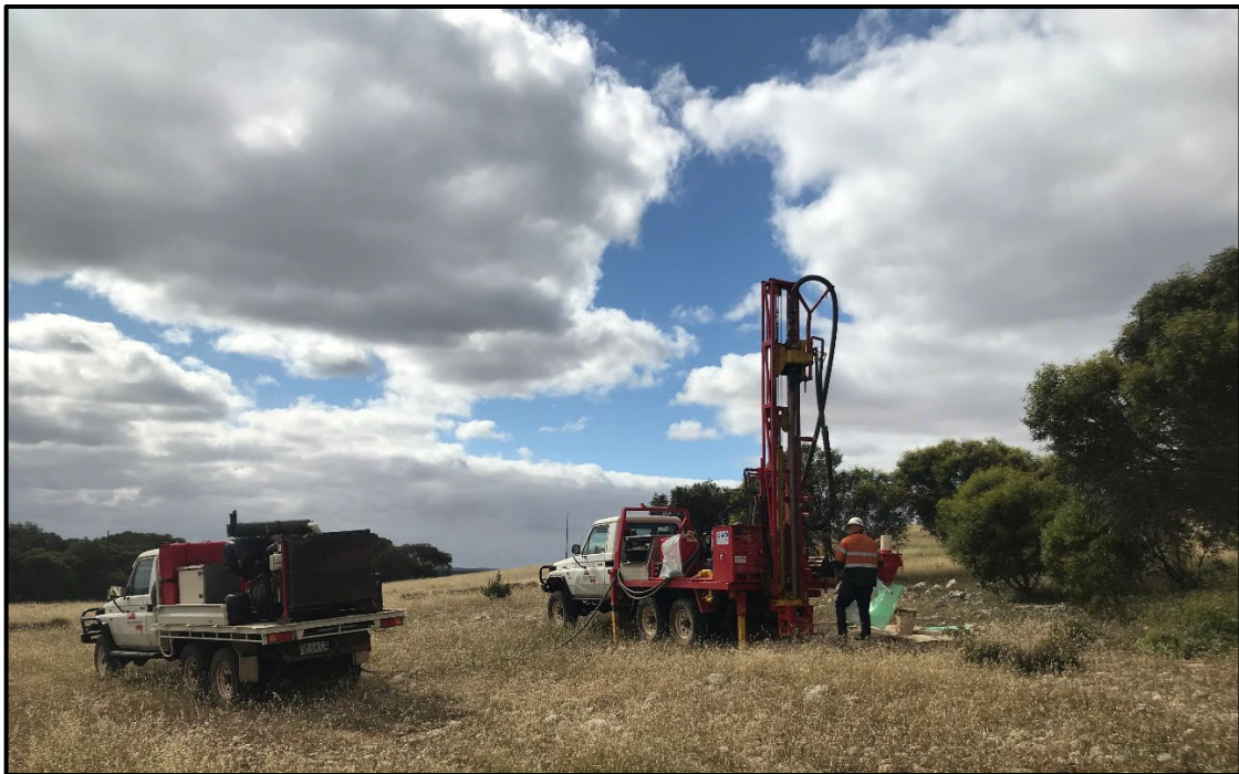
Figure 1: Air-Core Drilling at the Gibraltar Project (EL6506), South Australia
